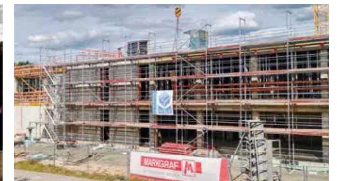
The construction site of the FZA
